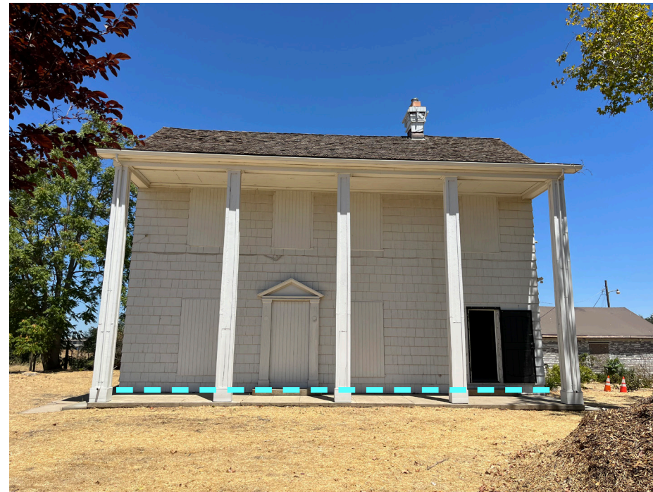
Figure 12: The front (south) facade of the Main House, view north (2024). Approximate location of new raised deck indicated by light blue dashed line.
