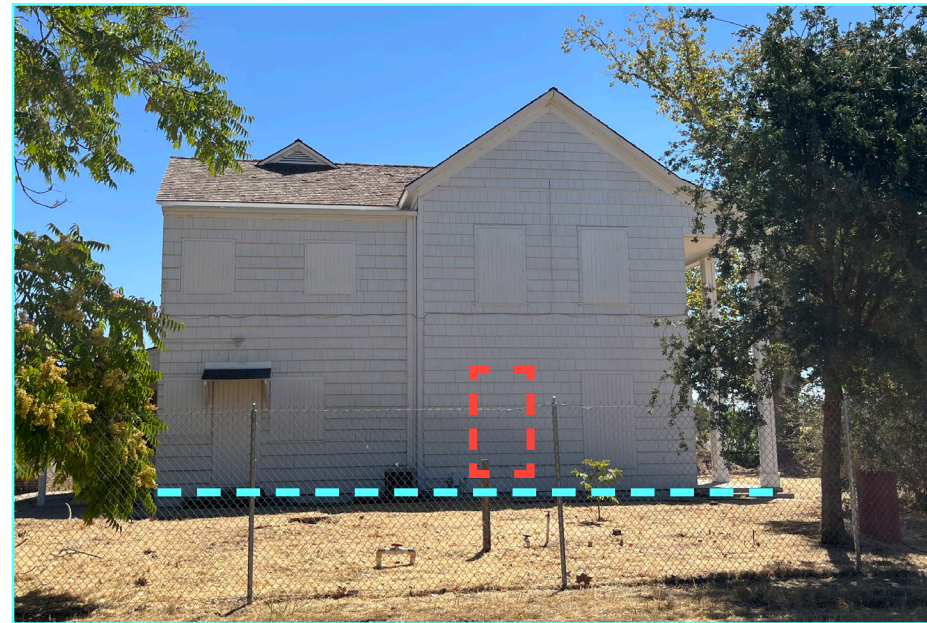
Figure 15: The west elevation of the Main House, view east (2024). The location of a window recommended to be reopened is outlined with a dotted red line. The approximate location of a new raised deck is indicated by light blue dashed line.
