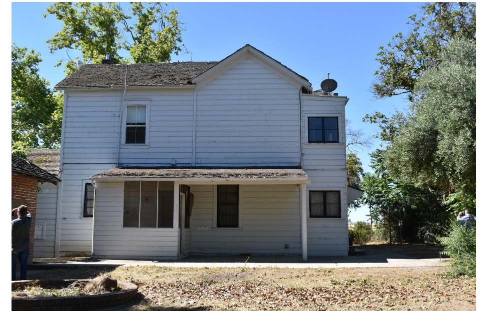
Figure 16: The rear (north) elevation of the Main House, view south (2017).
