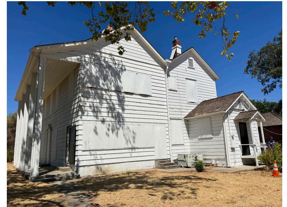
Figure 13: The east elevation of the Main House, view northwest (2024).
